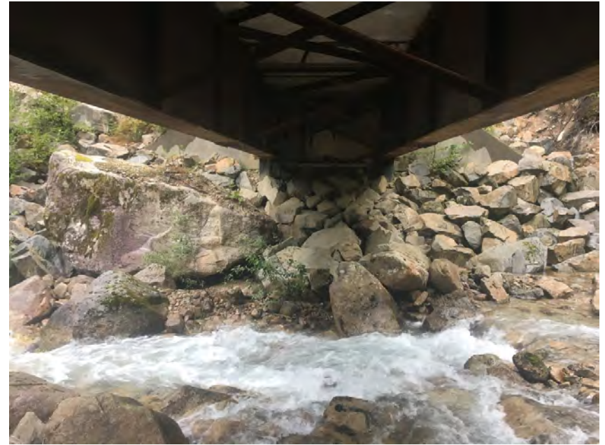
Right Bank Abutment when facing downstream
