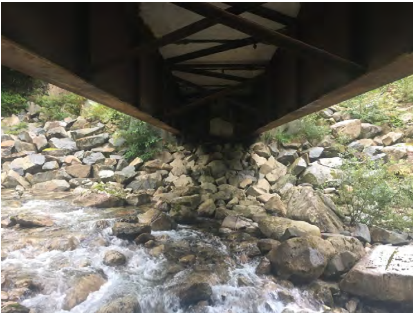
Left Bank Abutment when facing downstream
