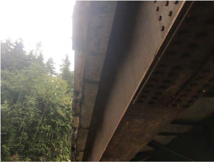
Deck panel bolts
